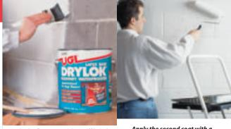
Apply the first coat with a stiff bristle brush working thoroughly into the pores of the masonry surface.
